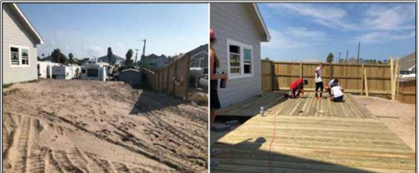
Before and after— the building of the rectory deck and surrounding fence
