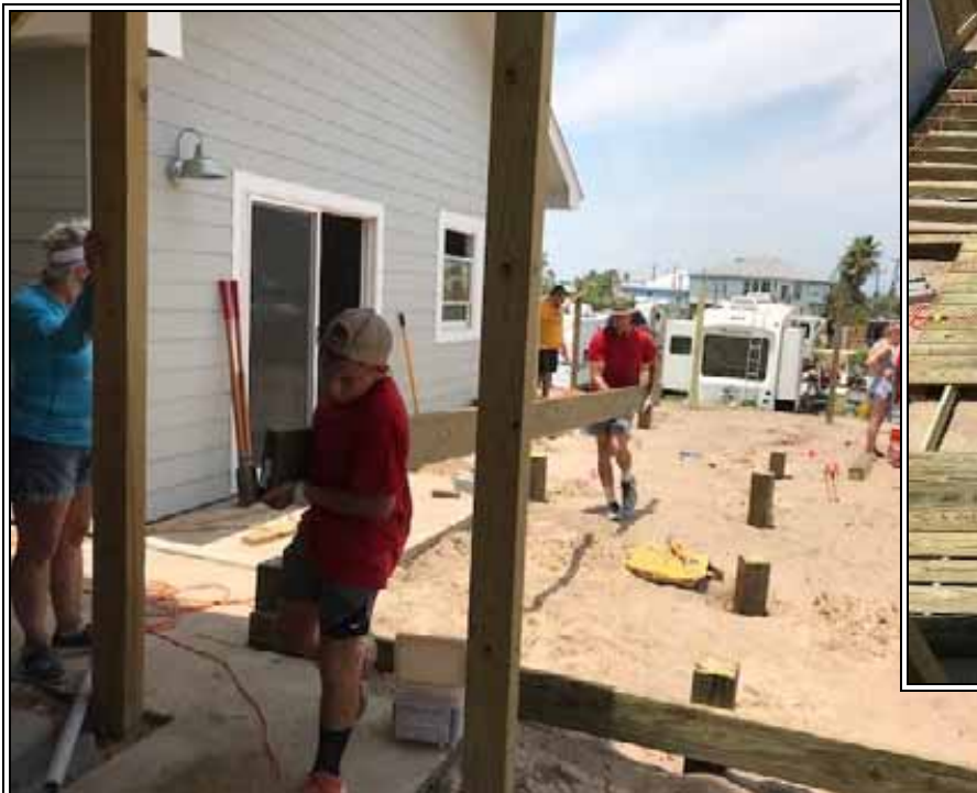
Beginning stages of building the rectory deck
